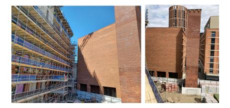
The wall is made of clay facing brickwork and is 17.93m high x 16.4m wide. It is 4.83m above ground level, with the overall height of the wall 22.6m high, <u>a drawing</u> of the elevation is available for download as a PDF.
